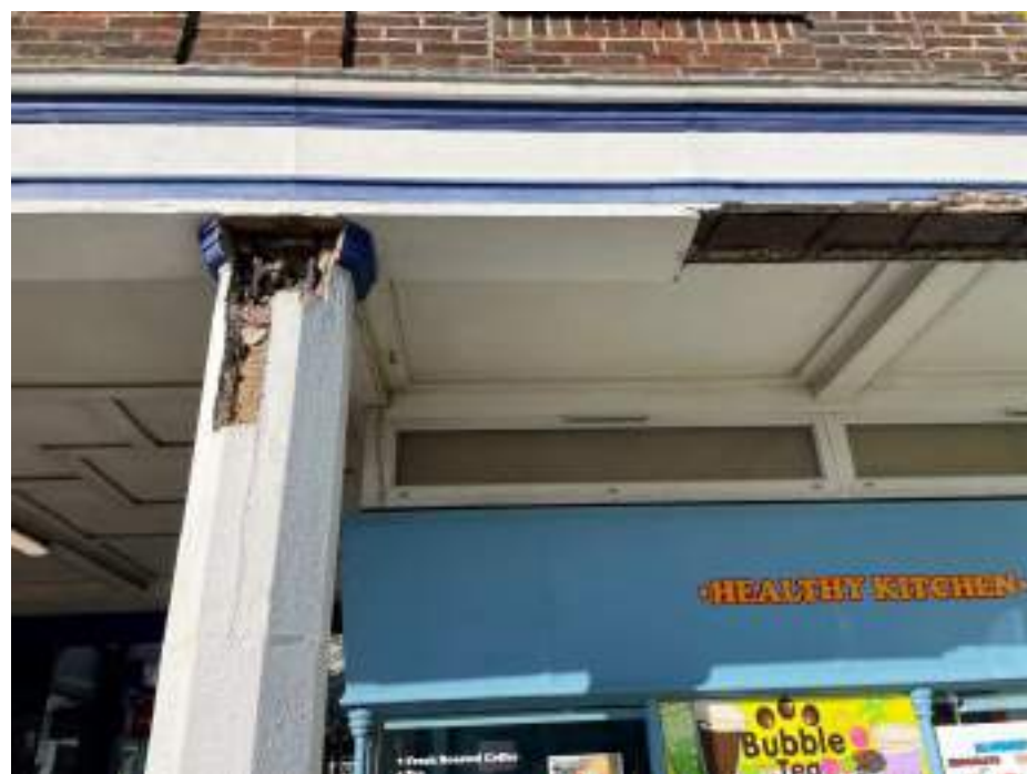
1. Exterior, Belmont Street
