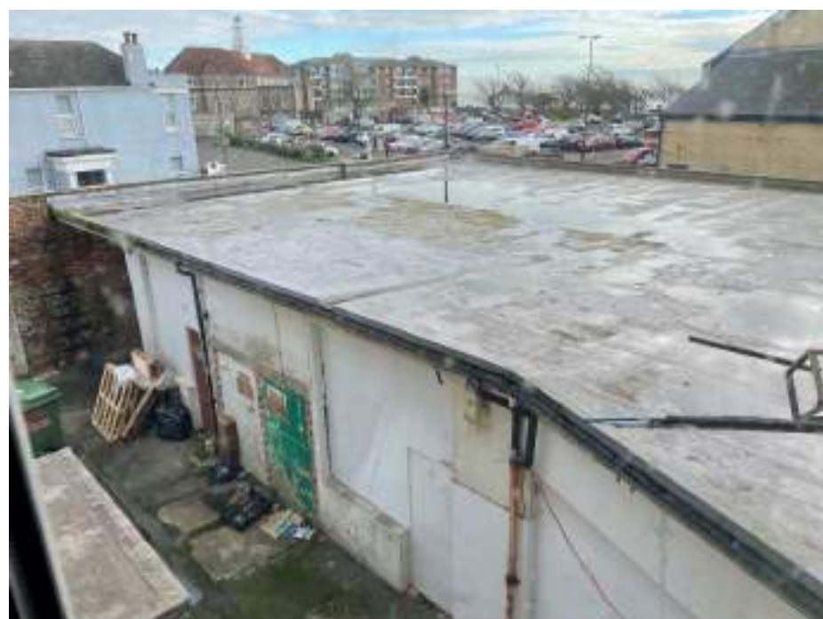
3. Exterior, roof over single storey unit on Belmont Street
